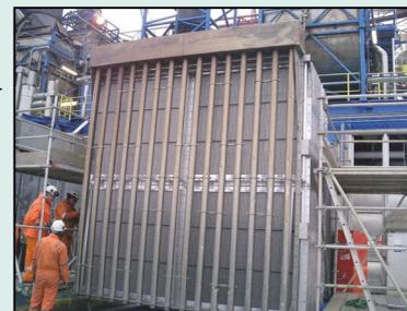
Statoil has since refurbished all of the main ventilation air intake housings on three other North Sea platforms with 19 new Infinidry filter units including over 700 Drop Safe pockets. The Infinidry System helped Statoil reduce operating costs, maintain higher air standards and led to some very happy machine operators.
