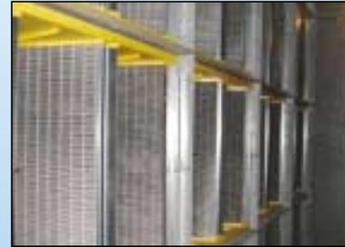
The Titan draws the air into the V and pushes it through the filter pack. Using this model, the air never hits the tips, as is very common with a standard 4-inch pleated filter.
